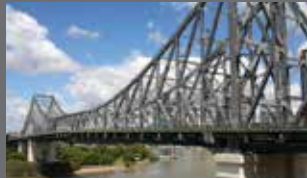
Steel bridge fabrication
