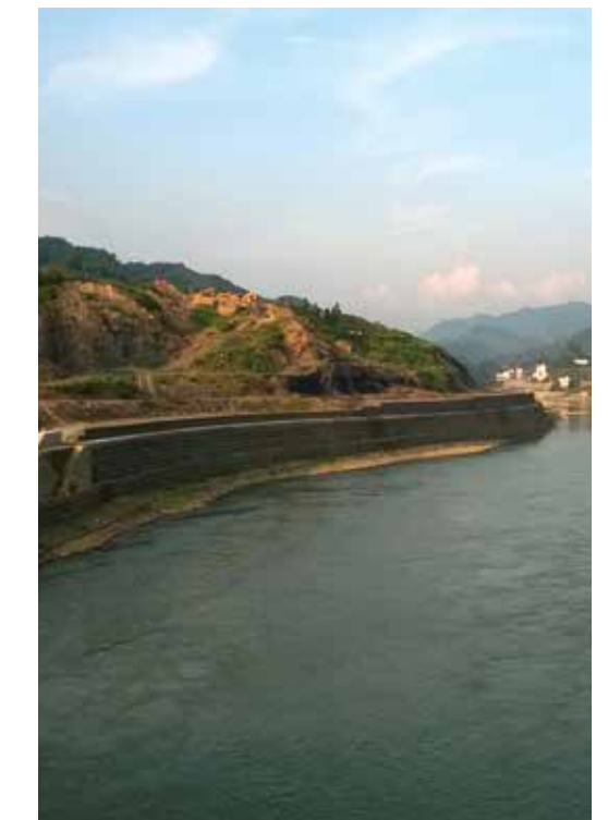
Longitudinal protection on major river
