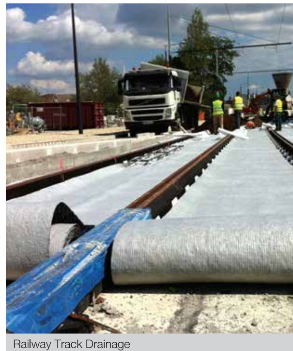
Railway Track Drainage
