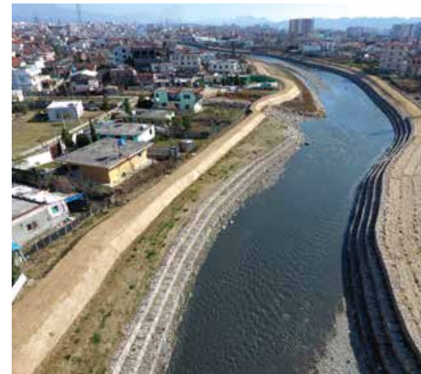
Channelling works containing river in urban area
