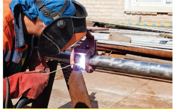
Stainless Steel Pipe Welding
