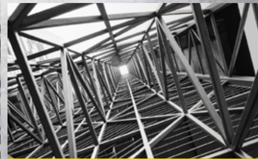
Structure and framework
