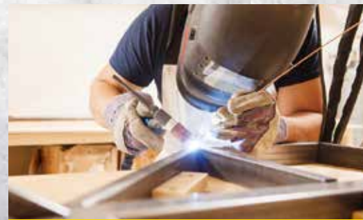
Stainless Steel Furniture Welding
