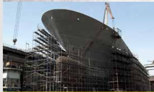
Ship body construction
