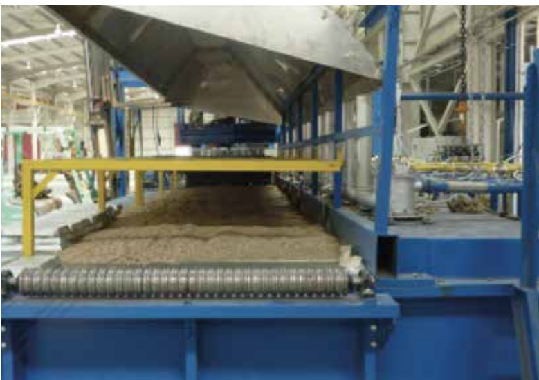
BSRM Production plant
